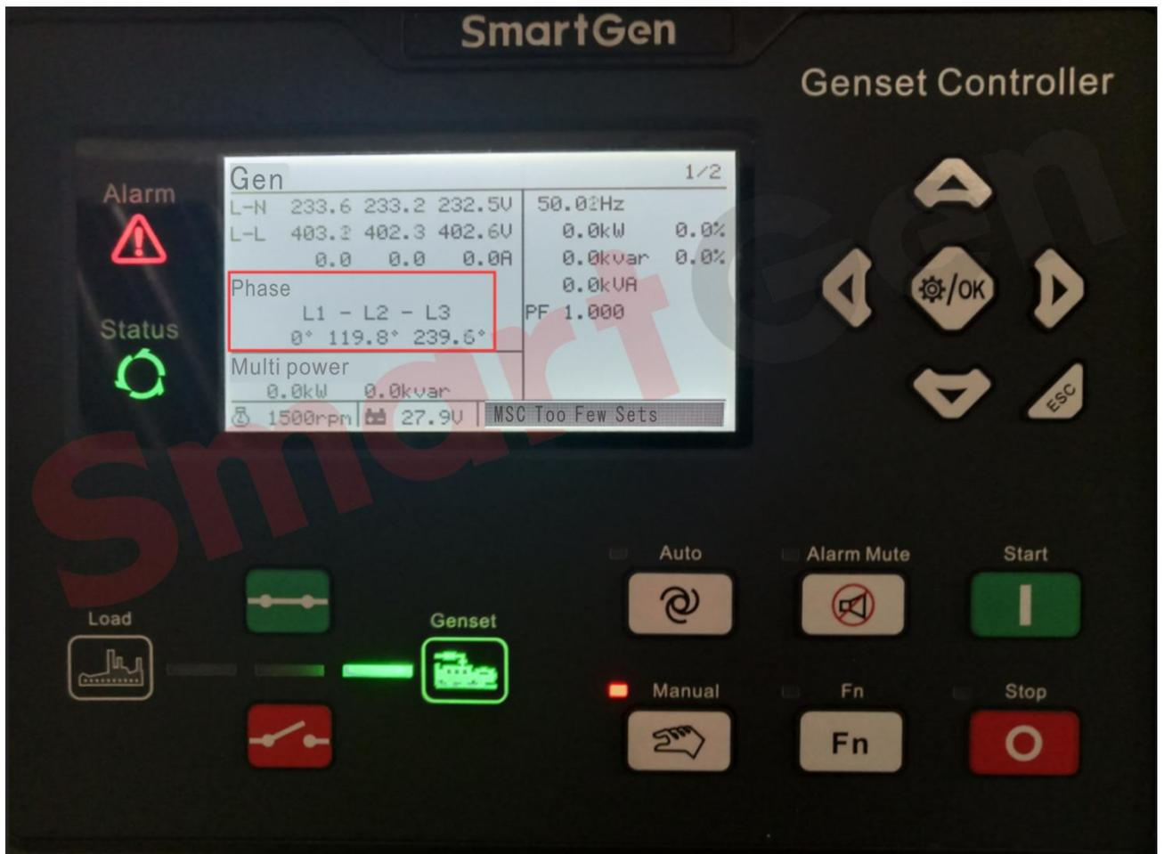
Fig.96 Correct phase sequence display
